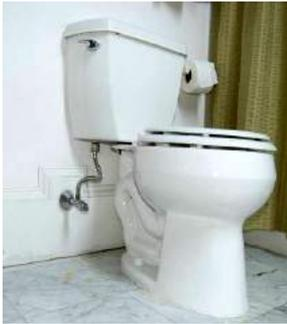
Figure 3: Flexible hose (Source: Picture by Iris D. Tommelein, Boston, MA, 2007)
