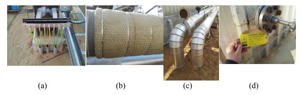
Figure 7: Cable Colour-Coding (a) and Pipe Insulation (b-c) with Instruments Attached (d)
