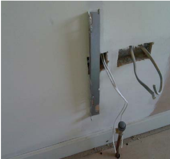
Figure 1: Hard clash on Site
