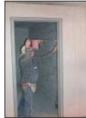
Figure 6: Drilling for Anchor Bolts
