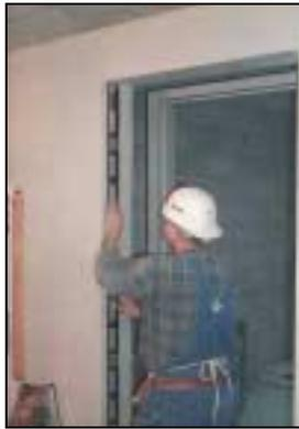
Figure 4: Drawing a Plumb Line
